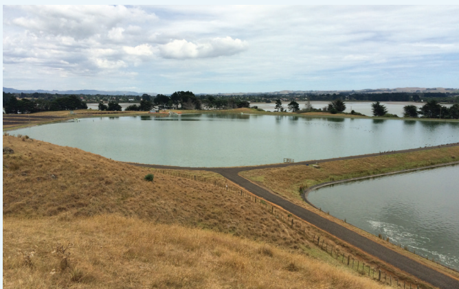
Waiuku Wastewater Treatment Plant.
