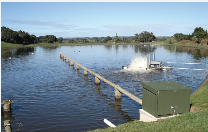
Clarks Beach Wastewater Treatment Plant.
