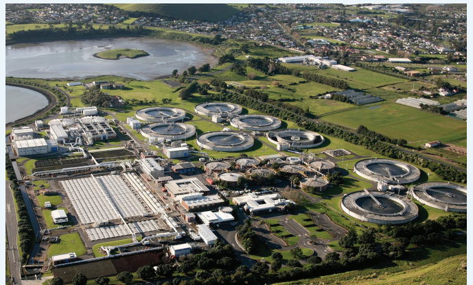
Mangere Wastewater Treatment Plant.
